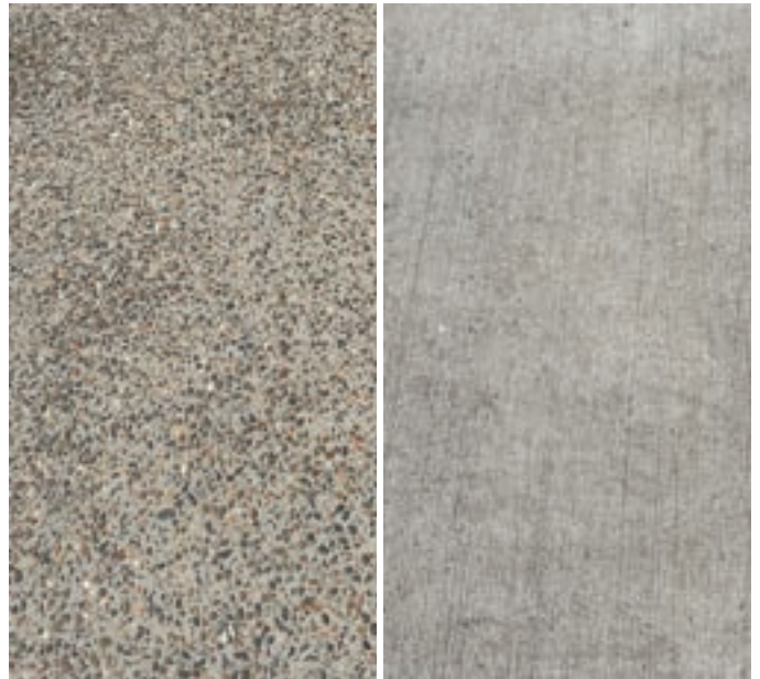
Sample -Concrete pavement (exposed aggregate finish (left) and broom finish (right))
