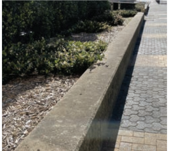
Sample - 400mm Wide Insitu concrete wall
