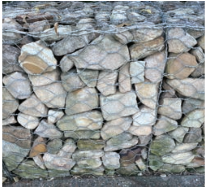
Sample - Gabion wall
