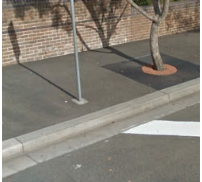
Sample - Insitu kerb & gutter - large size
