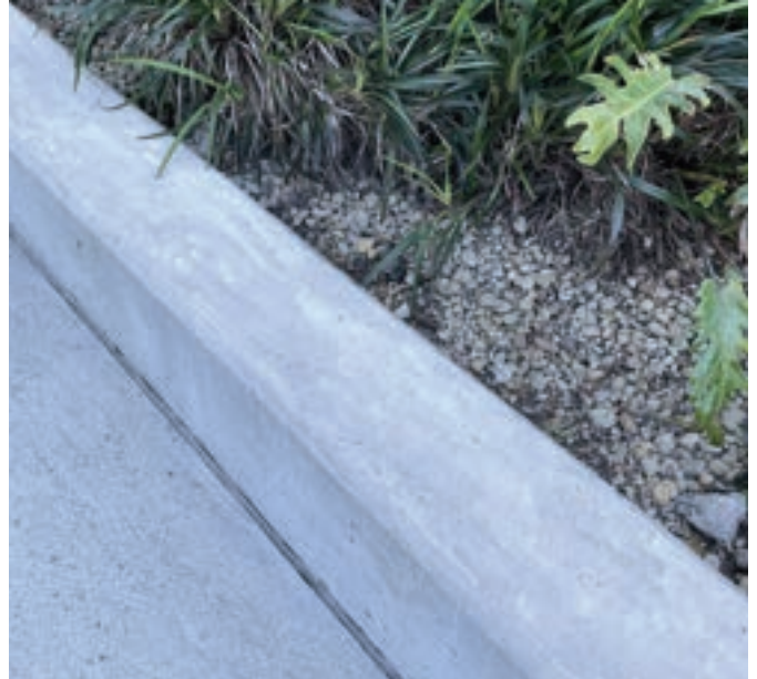
Sample - 200mm Wide insitu concrete retaining wall
