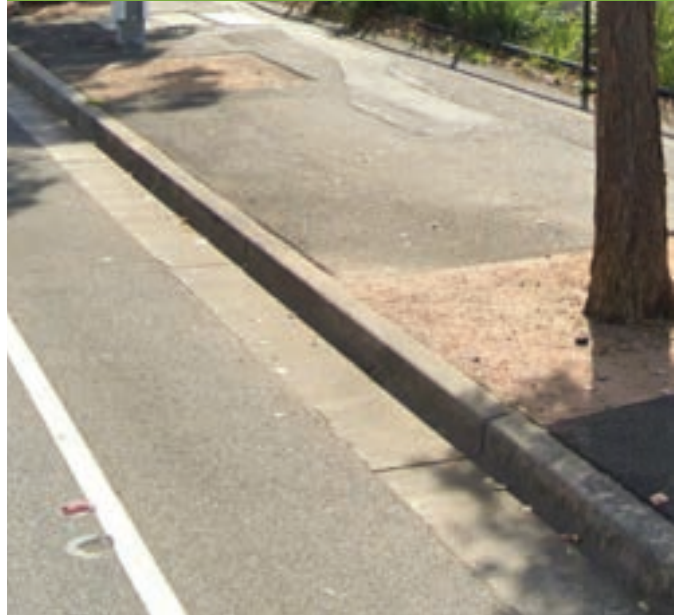
Sample - Insitu kerb & gutter - standard size
