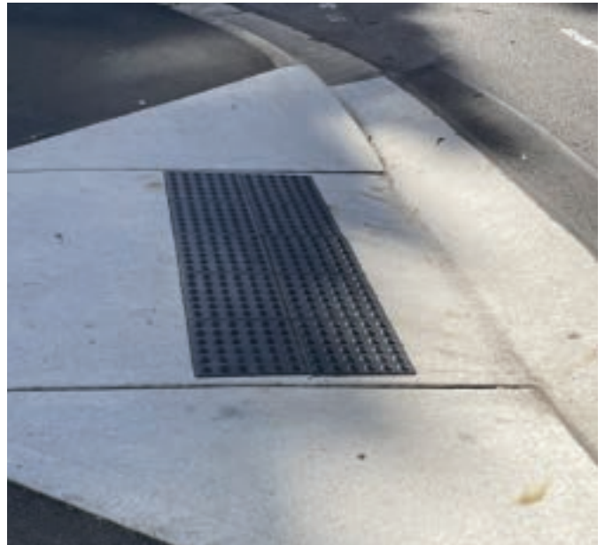
Sample - Standard kerb ramp
