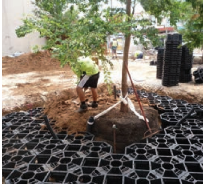
Sample - Tree planting with soil vault system
