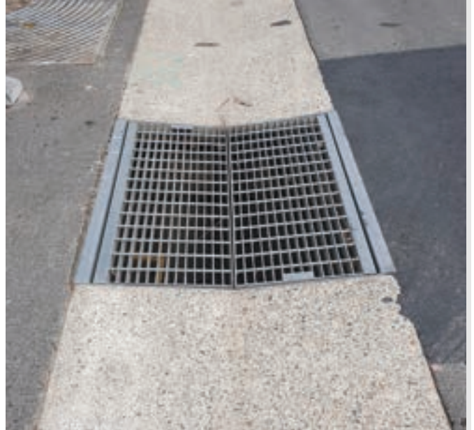
Sample - V-drain swale
