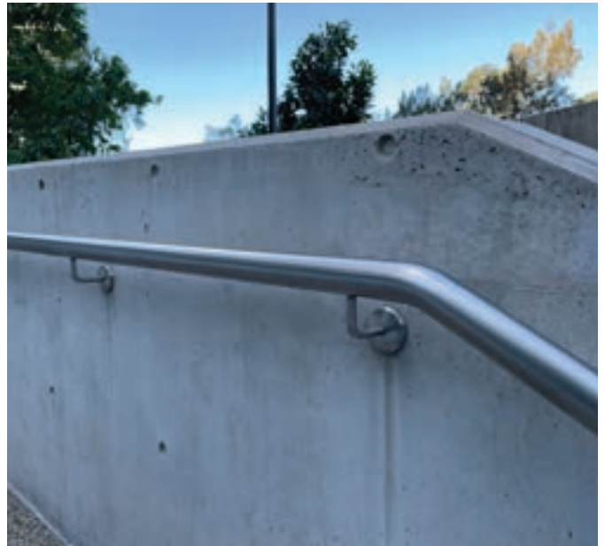
Sample - Handrail - wall mounted
